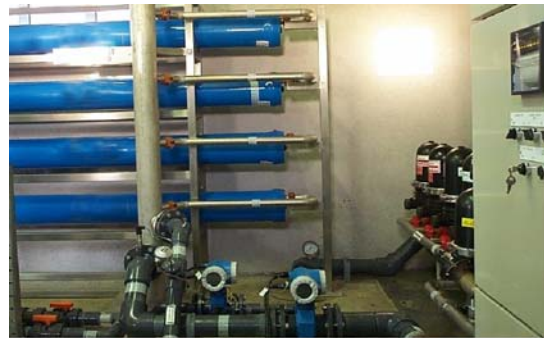
Ultra-filtration systems for drinking water treatment
