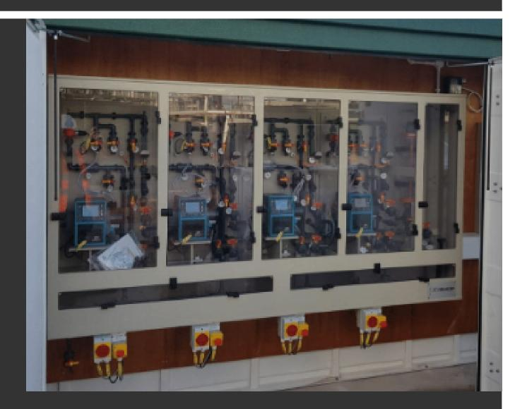
Each pump draws chemical from the storage tank through the common suction pipework. A flow switch installed on the outlet pipework in each pump compartment indicates if there is any flow from the pump. There is a pressure relief valve (set to 3.5 bar) on the pipework of each pump compartment.
